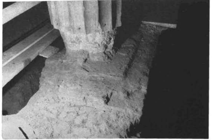
Fig. 195. S. Pietro in Vincoli, North colonnade, column 10, showing core of original base and square mortar seating
